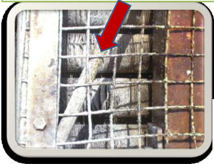
CALCIUM LAYER BEFORE CLEANING
